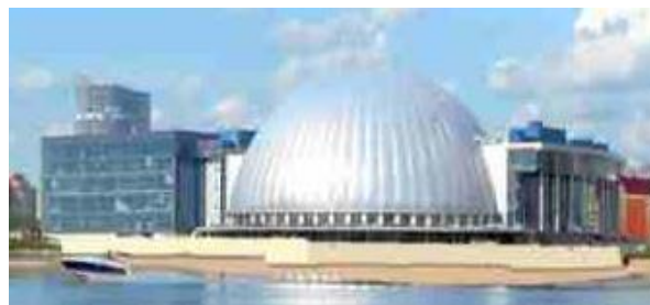
Figure 4 - «PITERLAND». One of the biggest wooden domes in the World with a 92 m diameter, SPb, RF, 2012
