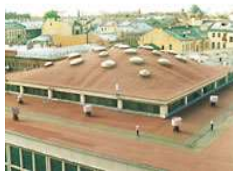
Figure 2 - Shallow reinforced concrete covering of the Nekrasovsky (Maltsevsky) market in St. Petersburg, 1960
