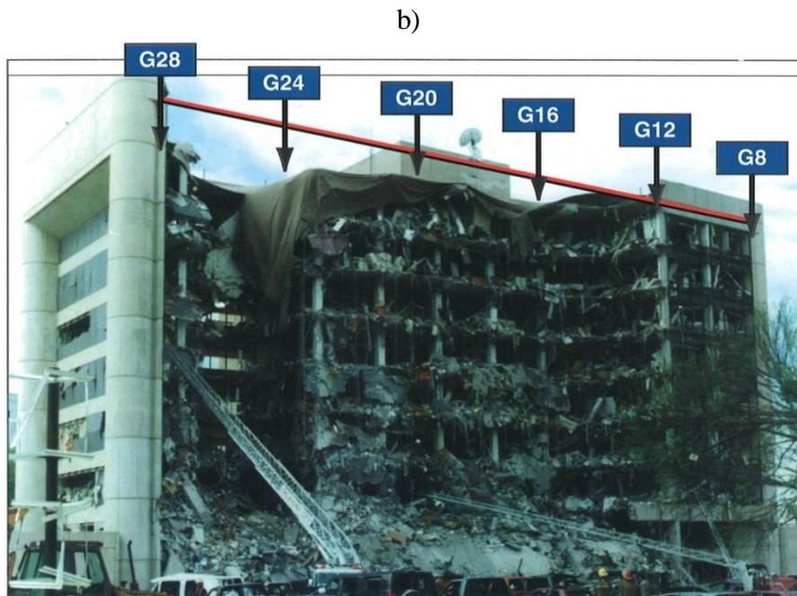
**Figure 1 - A picture of the collapse of a building by Alfred Murray, Oklahoma City, USA, 1995 [27]: diagram of the destruction of the structural structures of the building caused by the blast wave - a view from the side of the northern facade (a) general view of the eastern and northern facades of the building after the collapse (b)**
