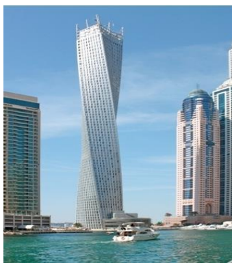
Figure 1 - Infinity Tower. Each side of it is a pseudo-developable helicoid
